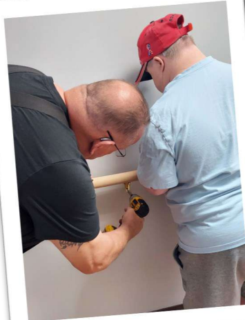
Eddie is assisting Duke with installing rails.
